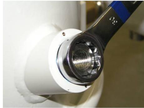
Installing a transducer
